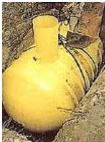
Cesspools are an ideal solution for locations where a septic tank cannot be installed, such as wet or poorly drained sites.
